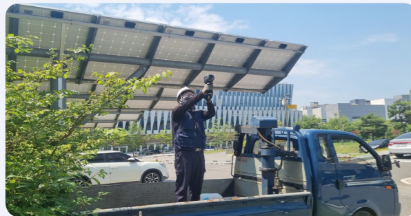
Safety Inspection of Solar Power Generation Facilities at Naju Building
