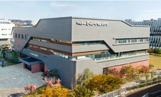
640, Bitgaram-ro, Naju-si, Jeollanam-do Combined Floor Area 4,295.50 / Four Stories: B1 to 3F Combined floor area: 4,295.5㎡ / B1 Electric Room, Machine Room, Document Room, Storage 1F Lobby, Office, Multi-purpose Hall / 2F Office / 3F Office, Lounge
