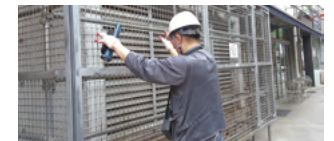
Fire Safety System Inspection at Daehakro Art Theater
