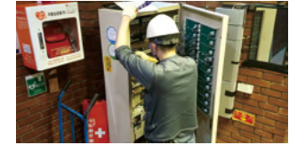
Fire Safety System Inspection at ARKO Arts Theater
